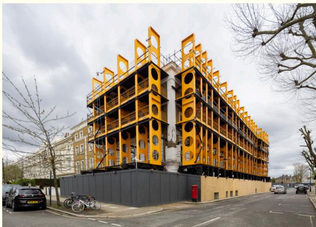
**1-7 QUEEN'S TERRACE:** At St John's Wood Square, McGee have installed a pioneering ribbon-cut modular facade retention system that is the first of its kind in the UK. This carbon-friendly solution represents a substantial reduction in carbon emissions as it can be taken apart and reused elsewhere after use.
